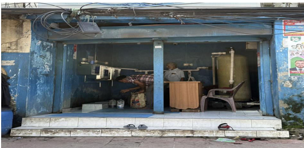
Fig. 1: Water Booth in Dhaka City.
